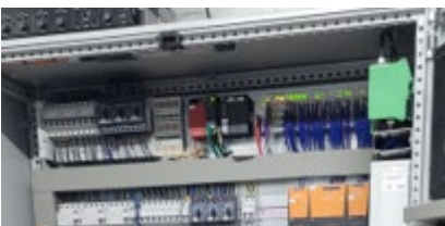
Pic 6: The MELSEC System-Q PLC control system manages all simulator functions
