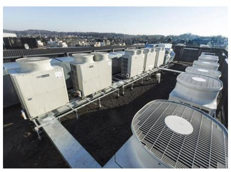
The VRF-R2 system moves otherwise unused heat into a part of the building where there is an actual need for heating or hot water.
