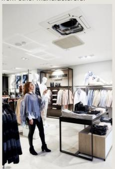
The filter cassette can glide down to 4 m in a matter of a few seconds.
