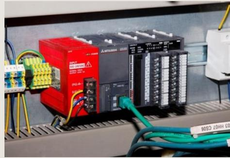
A FAG SmartController in the form of a Mitsubishi Electric PLC from the MELSEC L-series operates as a bidirectional gateway between the customer controller and sensors in the condition monitoring system. [Source: Mitsubishi Electric Europe B.V.]
