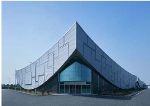
Picture 1: Changshu Innovation Centre for Green & Intelligent Manufacturing, China.
